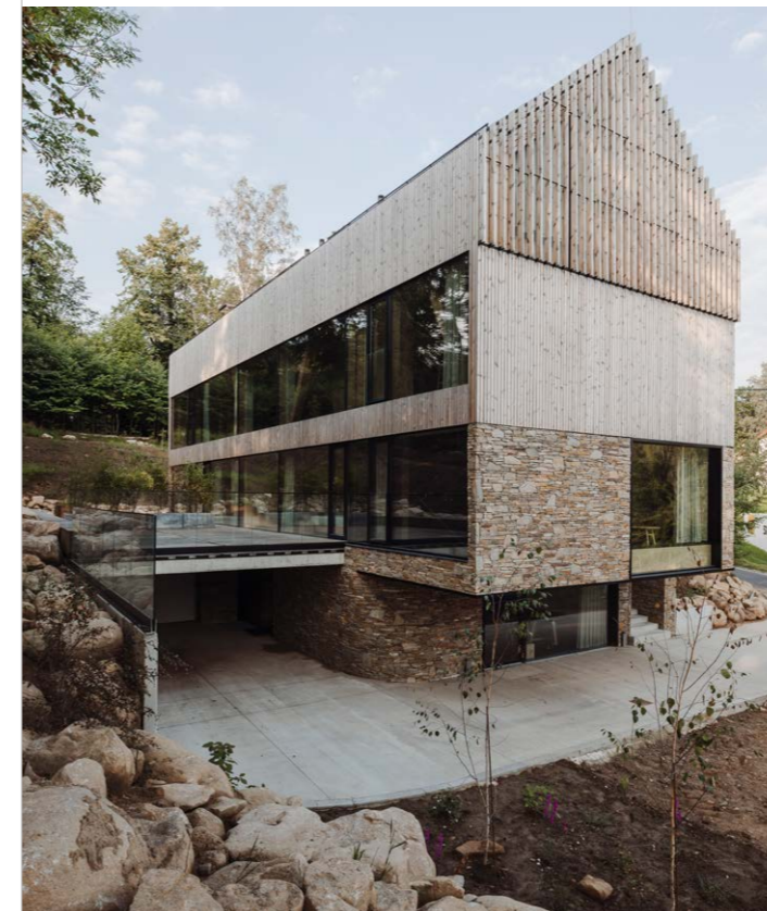
Uncoiled Benchmark thermo-pine cladding and roofing one year after installation. Apartments in Poland Photo and distribution: Komplex Market
