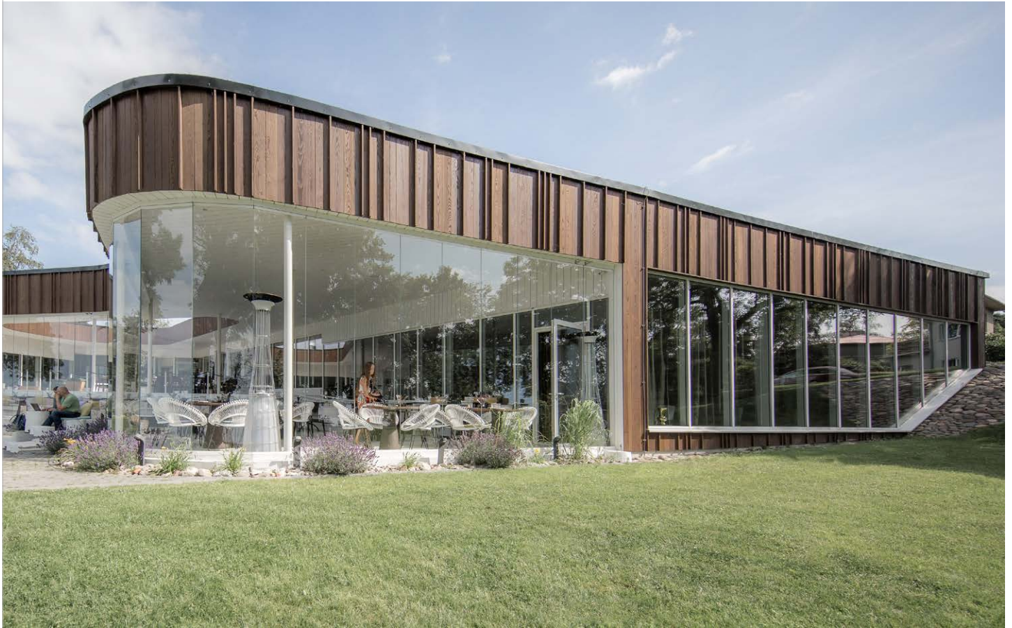
Oiled Thermory Benchmark thermo-ash cladding. NOA Restaurant in Estonia Photography Elvo Jakobson
