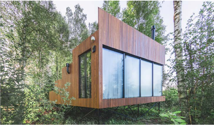
Thermory Benchmark thermo-ash cladding few months after installation. Maidla Nature Resort in Estonia Photography Elvo Jakobson
