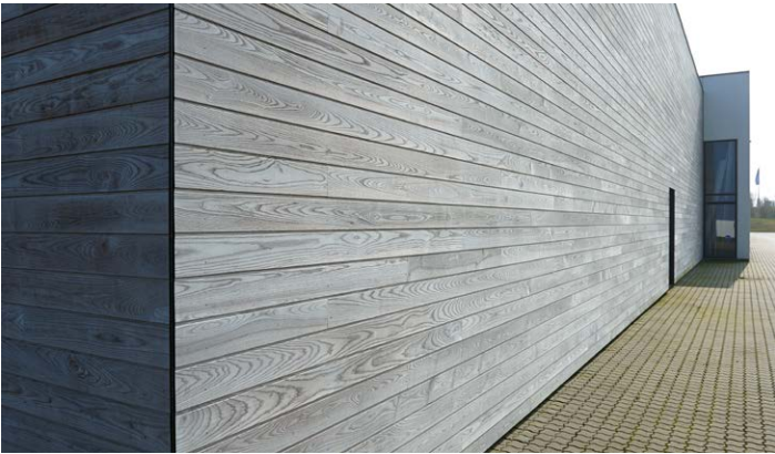
Unoled Thermory Benchmark thermo-ash one year after installation Denmark
