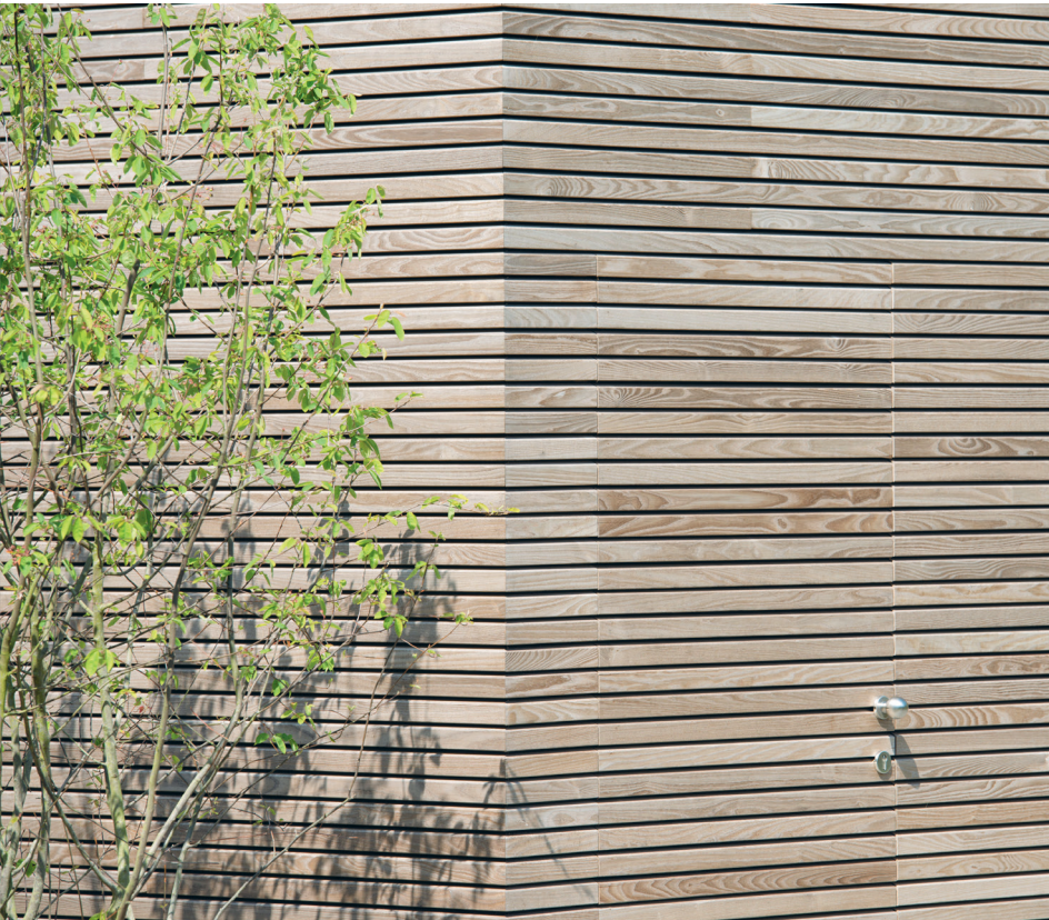
Cut the boards to a 45-degree angle.
