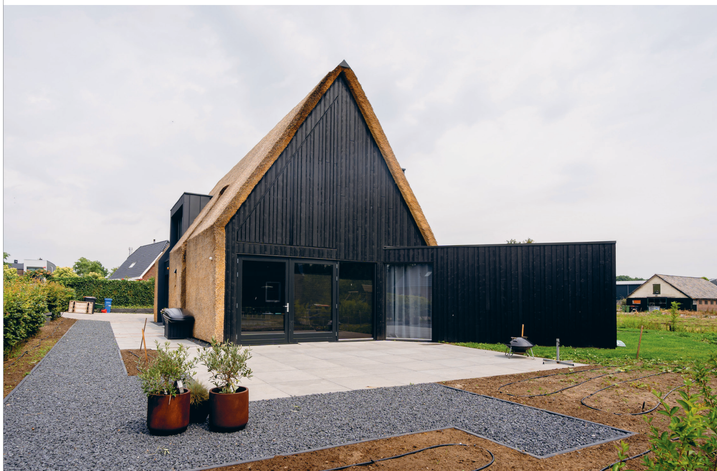
Vivid by Thermory thermo-spruce cladding (D4 / Channelsiding), color Black. Private house in Netherlands. Distribution & Photo by InterFaca
