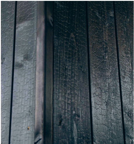
Corner profile: CP3. Painted on site
