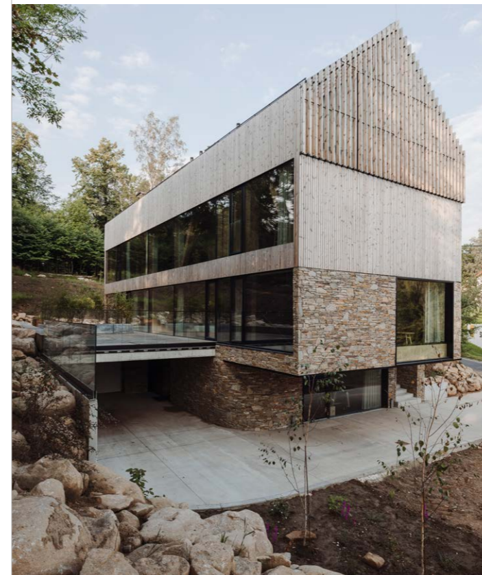
Uncoiled Benchmark thermo-pine cladding and roofing one year after installation. Apartments in Poland Photo and distribution: Komplex Market
