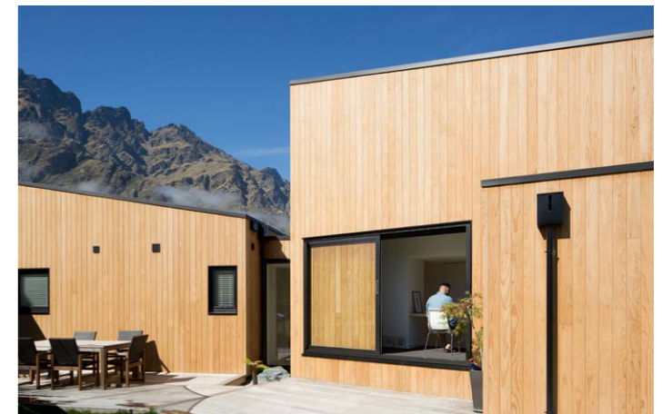
Benchmark thermo-radiata pine cladding. Jack's Point House in New Zealand Photography Sarah Rowlands Photography
