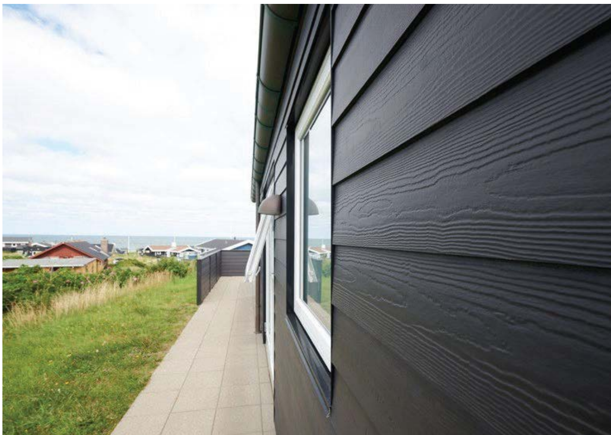
Hardie® Plank - horisontal montering med overlapping. Farge: svart
