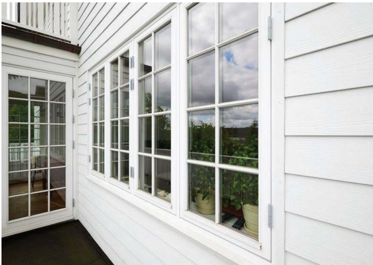
Hardie® Plank - horisontal montering med overlapping. Farge: hvit
